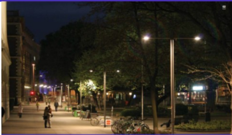
Public lighting, Vienna (Photo: City of Vienna)
